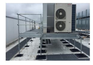
The air-handling unit frameworks had to achieve specific target heights of 800mm and 1000mm in height above the finished roof level, whilst also contending with a 2-degree roof fall. Pump House supplied purpose made leg assemblies with their heavy duty Flexi-Frames to achieve these specific project requirements.
