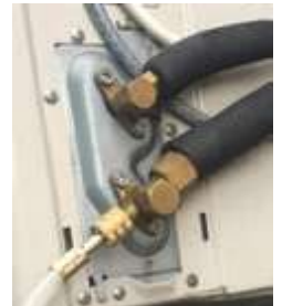
5. Connect the hose fitting only to the low pressure service point.
