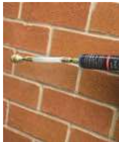
2. Remove syringe cap and connect the hose.
