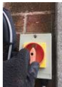
6. Turn system on and immediately inject the product when the suction pressure is at its lowest.
