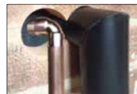
4. FIT THE ELBOW OVER THE COPPER PIPES.
