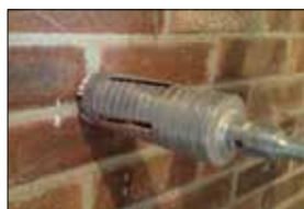
1. SELECT A 65MM CORE DRILL.
